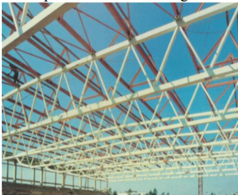
(a) Roof with lattice girders
