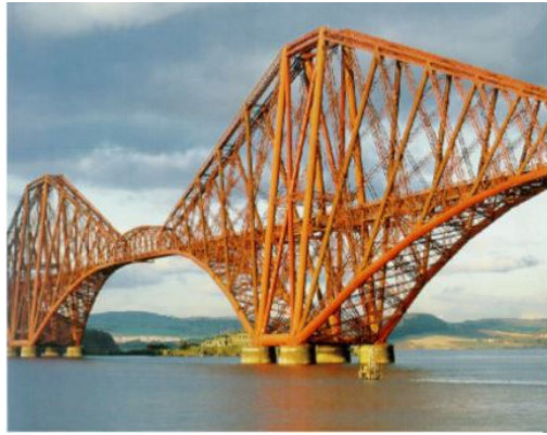
(c) Firth of Forth Bridge
